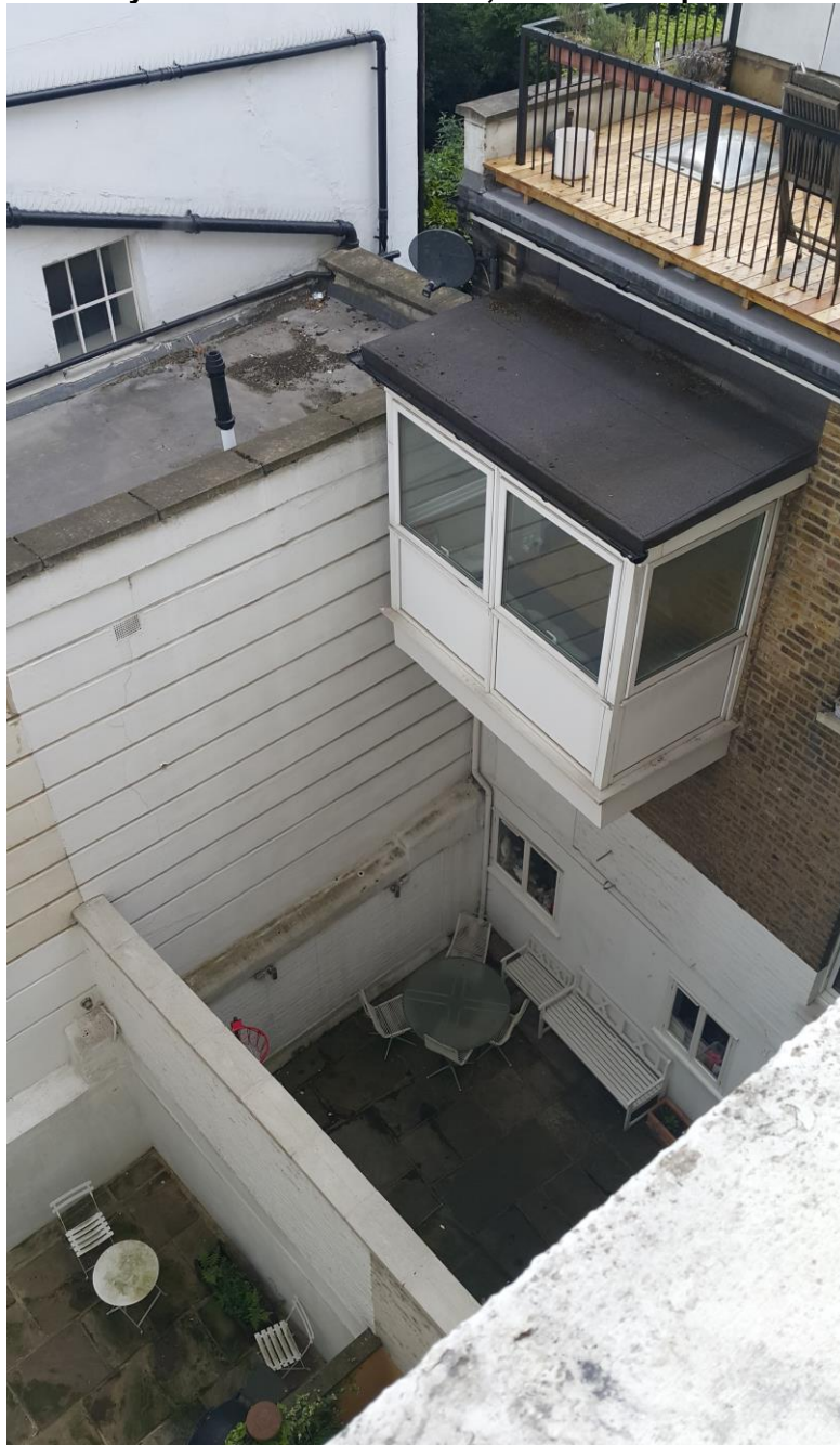
View of Courtyard from Second Floor, No. 1 St Stephen's Crescent
