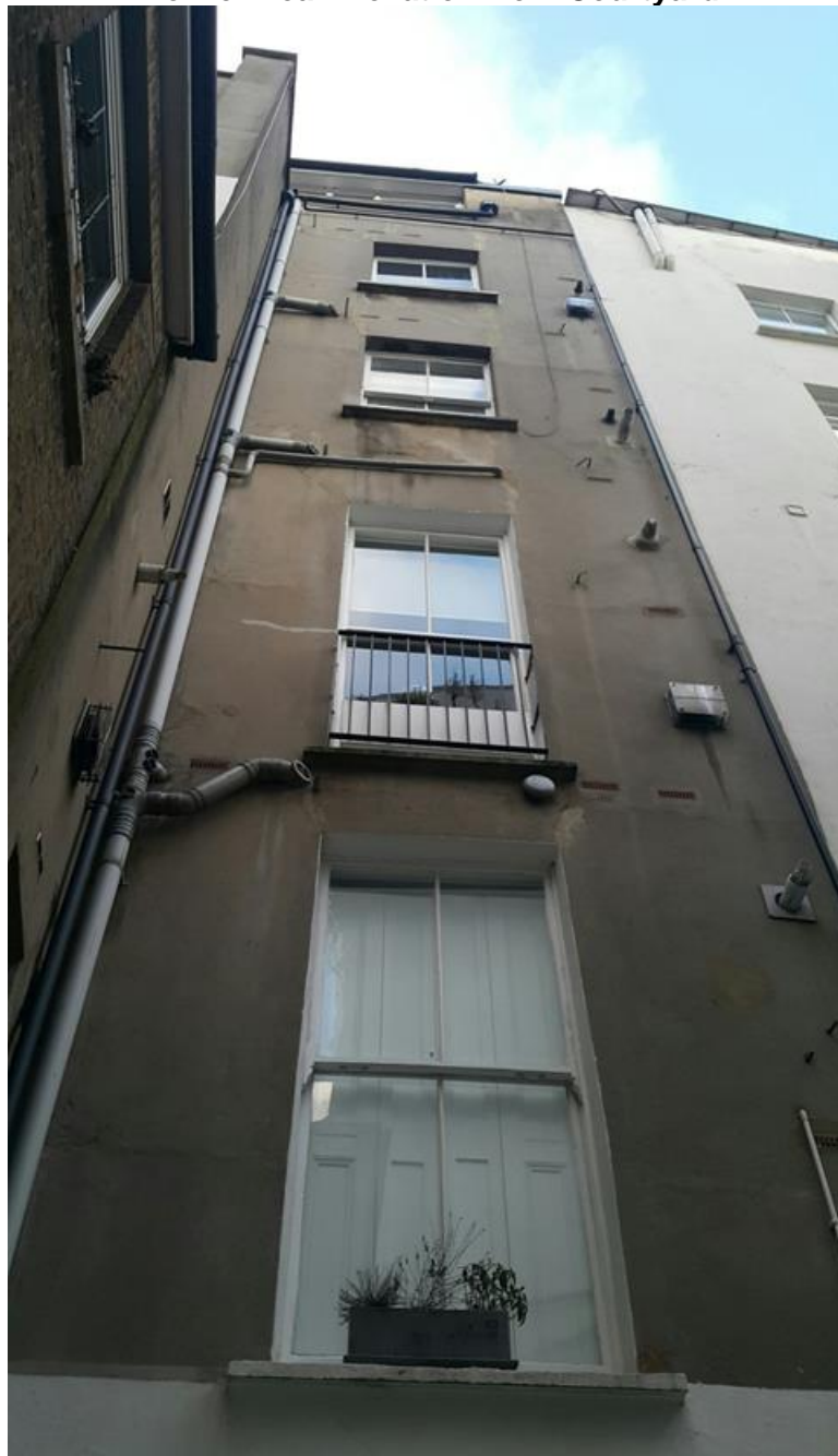
View of Rear Elevation from Courtyard
